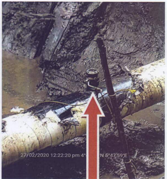
AFTER EXCAVATION (SPILL POINT)
